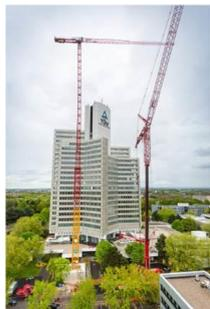
Heavy equipment: The WOLFF was assembled to its full height in only 2 ½ days with a 750 ton mobile crane.
